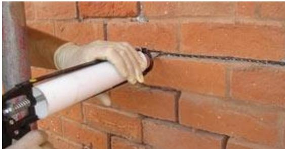
The bed joint can then be re-pointed in colour matched mortar.
